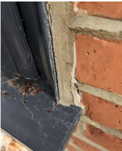
POINTING RENDER Lose mortar bottom right or window
