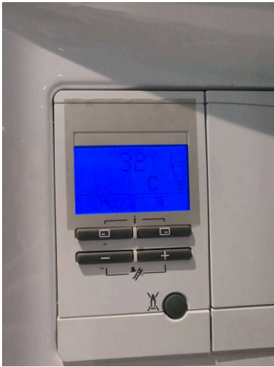
BOILER AND PRESSURE GAUGE
