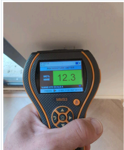
METER IN POSITION
