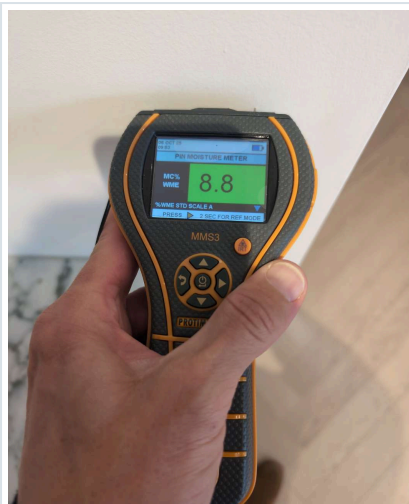
METER IN POSITION
