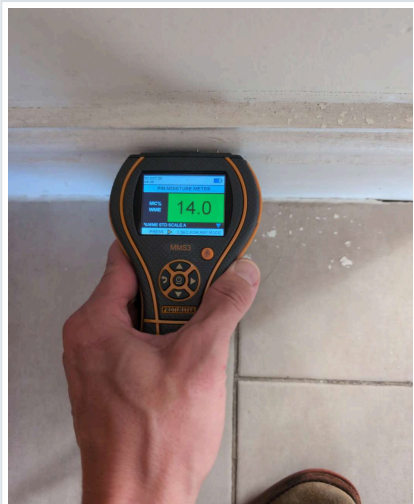
METER SHOWING THE READING
