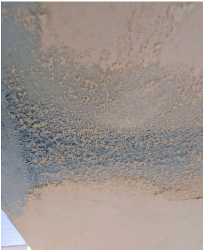
DEFECT Blue staining along a metal corner bead, with salts on the surface
