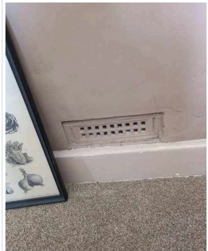
OTHER Chimney breast vent
