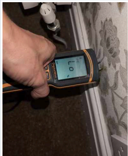
OTHER North external wall
