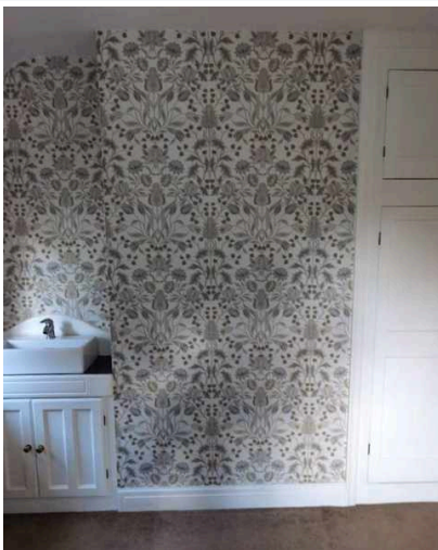
OTHER Chimney breast, sealed
