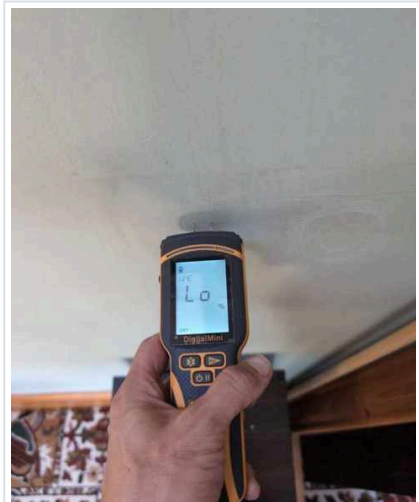
OTHER East external wall
