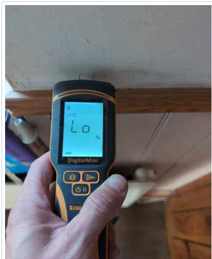
OTHER East external wall
