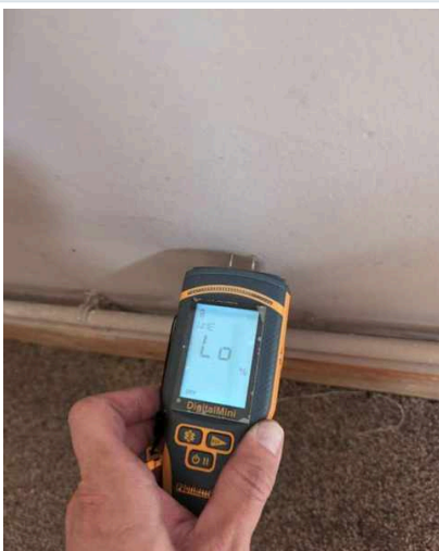
OTHER East external wall
