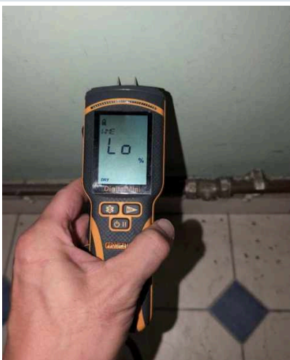
OTHER East external wall
