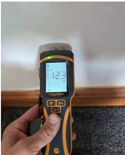
OTHER North internal partition wall
