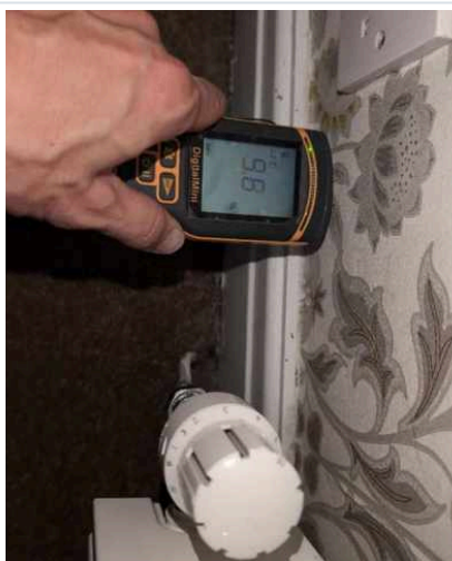
OTHER North external wall
