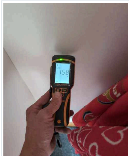
OTHER North internal partition wall
