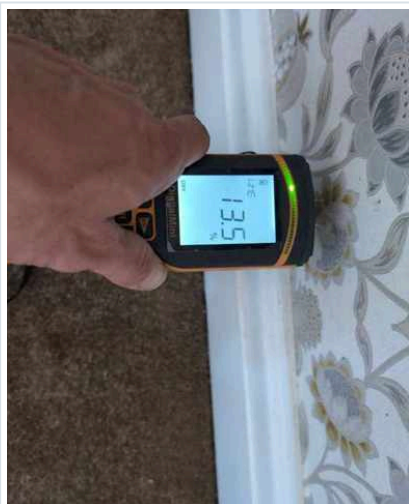
OTHER East external wall
