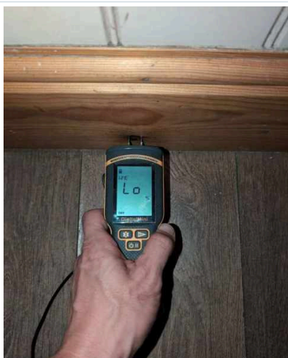
OTHER North external wall
