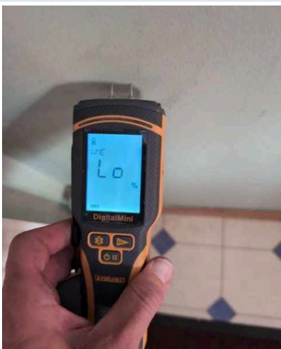
OTHER North external wall
