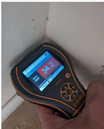
METER SHOWING THE READING
