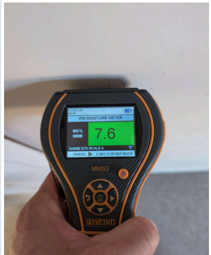
METER IN POSITION
