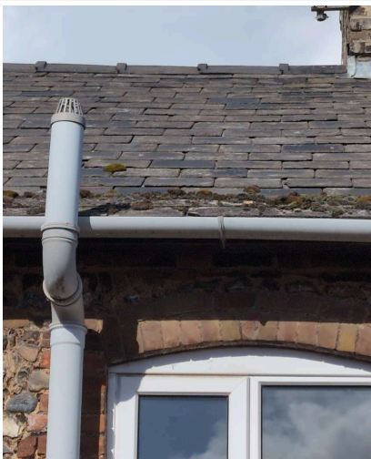
ROOF VISIBLE Rear roof slope
