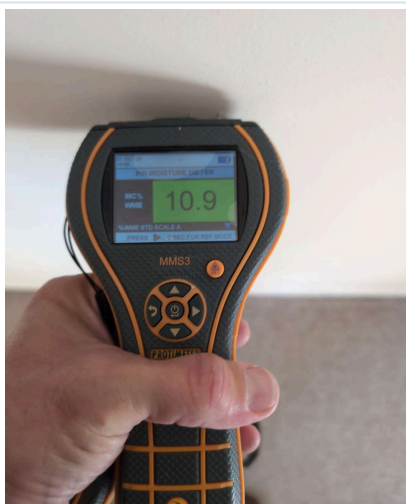
METER SHOWING THE READING
