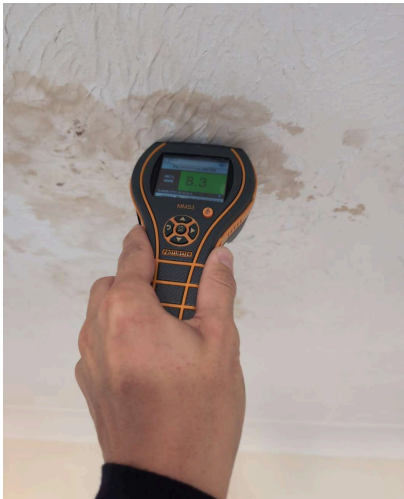
METER SHOWING THE READING
